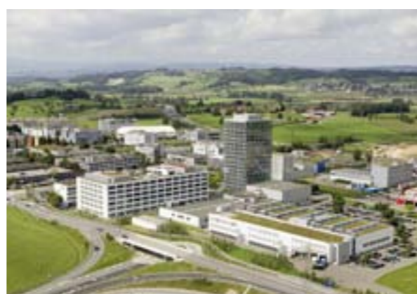
Roche Diagnostics International AG, Rotkreuz 26
